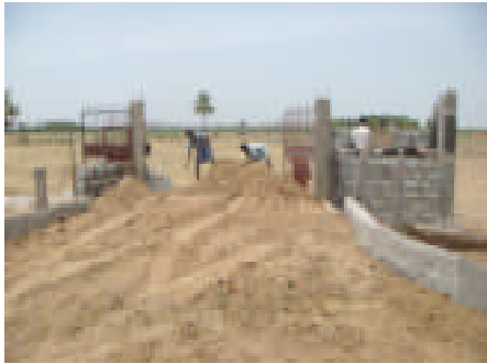
Illustration 4. The soil, which had to be added at the main gate to level the land with the road.
