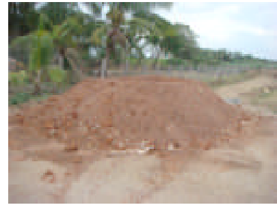
Illustration 7. The soil for the temporary water tank.
