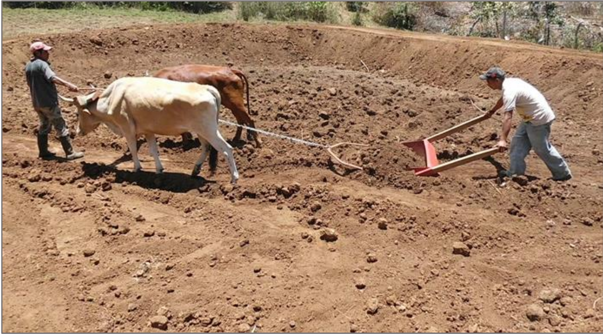
Illustration 25: Farmers working at the construction of the Pelón reservoir. Source: R.A., iDE Honduras, 2014.
