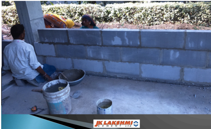
Figure 2: Indian Cement Firm constructs LC3 blocks for the Swiss Embassy in India. Source: Saxena
