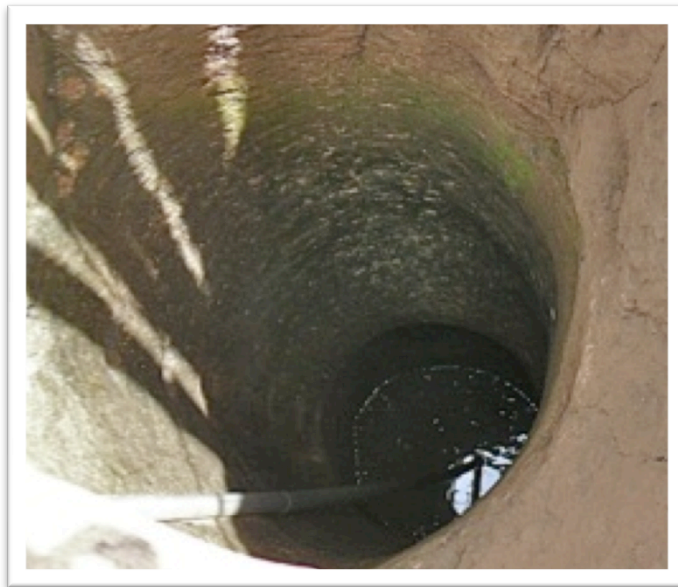
Figure 16: Well without lining ( Source: Own figure )
