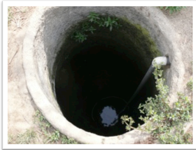
Figure 15: Lined well ( Source: Own figure )
