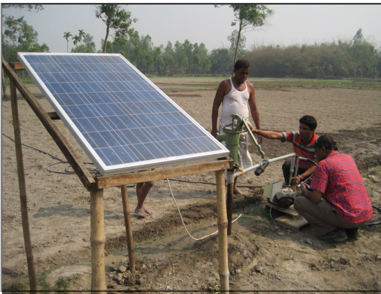
Micro solar water pump and solar panel
