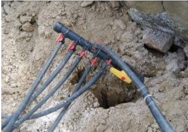
Distribution system from sub main to the laterals with various valves
