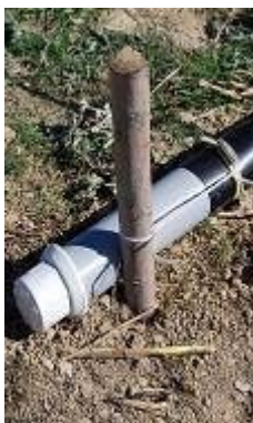
Picture 21: tied PVC flush valve in the field
