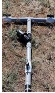
Picture 18: PVC tee connector set in between a filter and valves leading to the sub mains
