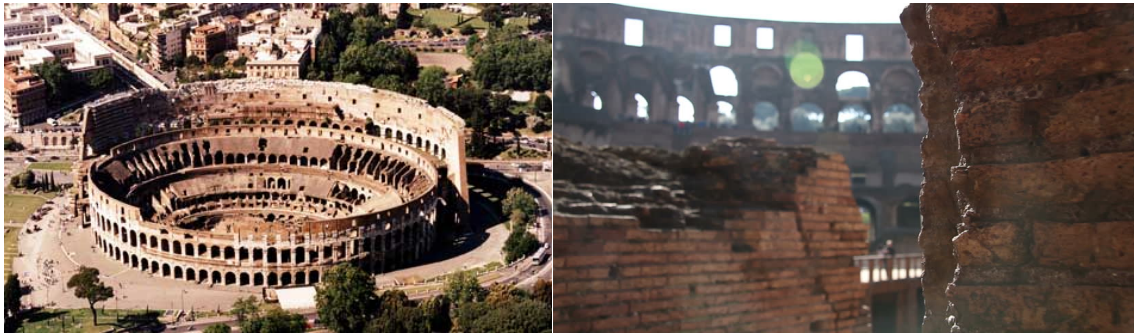
Figure 22: The Colosseum in Rome was made with a high proportion of bricks
